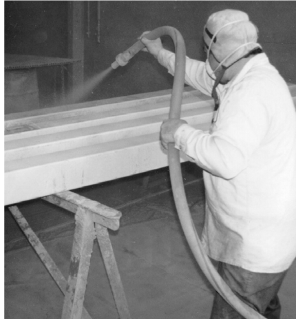
Fig. 6 - Sweep Blasting of Galvanized Steel Surface
